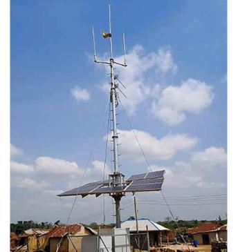
enabling relay hops of wireless signals to distances of over 40 km, overcoming both distance and — with NLOS tech — barriers like buildings, mountains, and trees.
